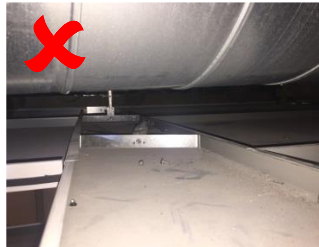
Example: Cable bundles resting/load ing on the ceiling
