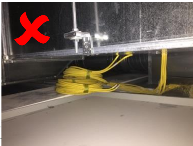
Example: Cable bundles resting/load ing on the ceiling
